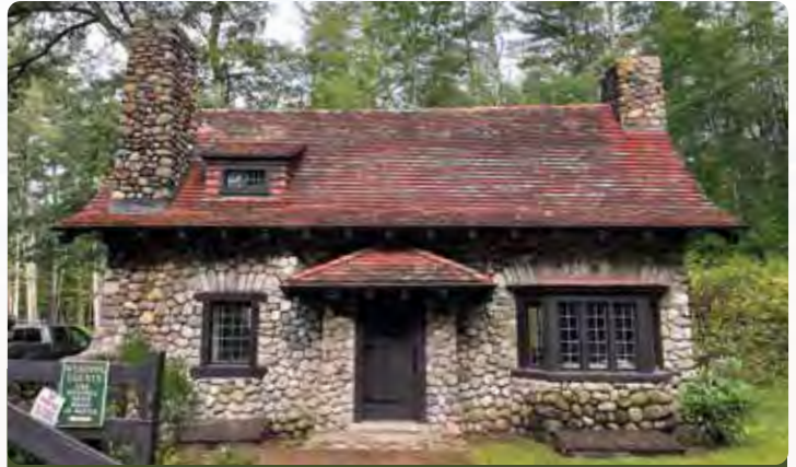
Brook Lodge interior rehabilitation to commence soon!
